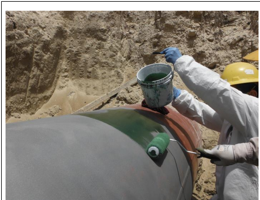
Fig. 6 – Application of Epoxy 314™ in the area to be repaired.
