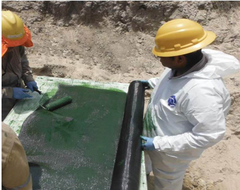
Fig. 7 – Use of a table for impregnation of Carbon 12K™ fiber with Epoxy 314™ .
